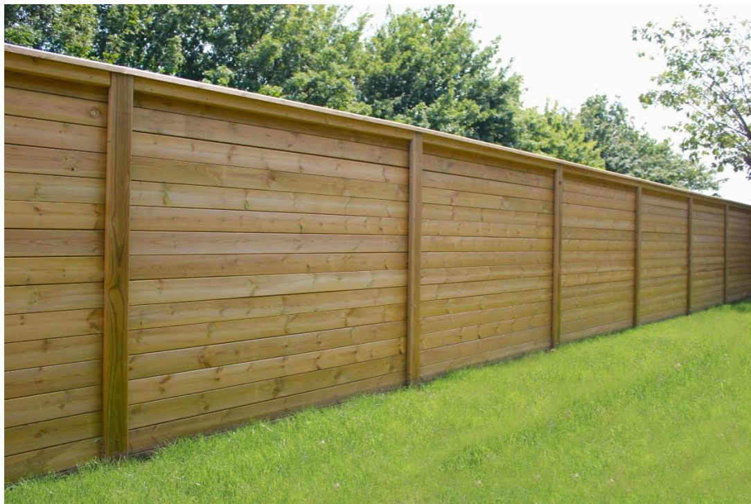
Fig 79. Illustrative example of the use of close boarded acoustic timber fencing
