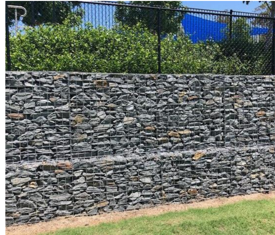
Fig 80. Illustrative example of the use of stone filled gabion baskets to act as an architectural solution for an acoustic barrier
