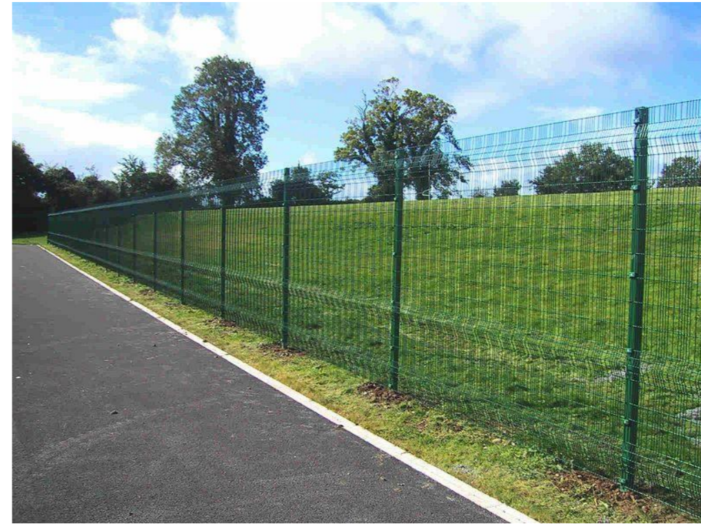
Fig 77. Illustrative example of 2.4m high paladin security fence
